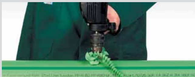
Drilling through the pipe wall
