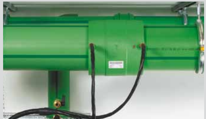
Adjust the socket diameter on the welding device. Start and control welding process. Keep the cooling time. Finished!
