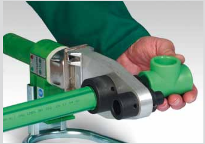
Heating-up of pipe and fitting
