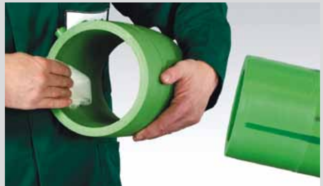
Clean the inner surface of the electrofusion socket
