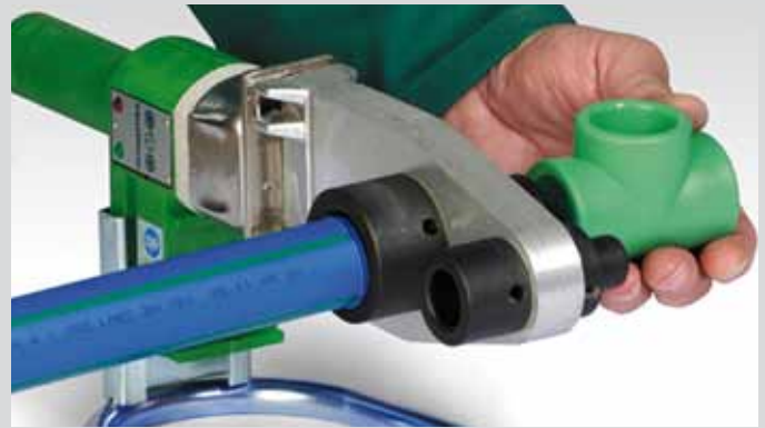
Heating-up of pipe and fitting
