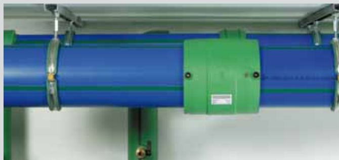
Push the second pipe - also peeled and cleaned - into the socket
