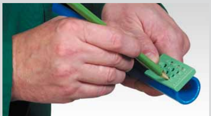
Marking of the welding depth
