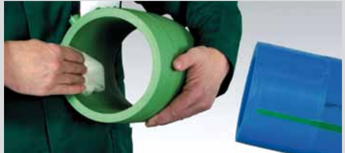
Clean the inner surface of the electrofusion socket
