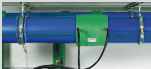
Adjust the socket diameter on the welding device. Start and control welding process. Keep the cooling time. Finished!
