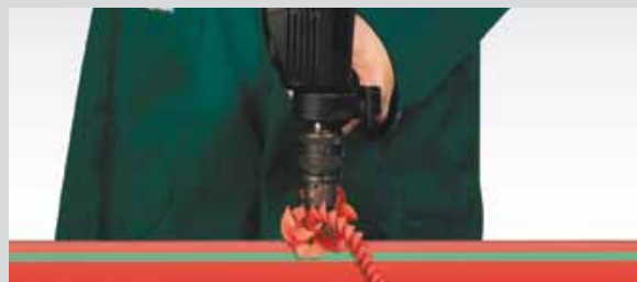
Drilling through the pipe wall
