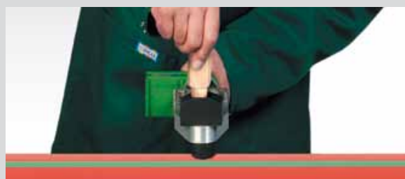
Heat-up of pipe...
